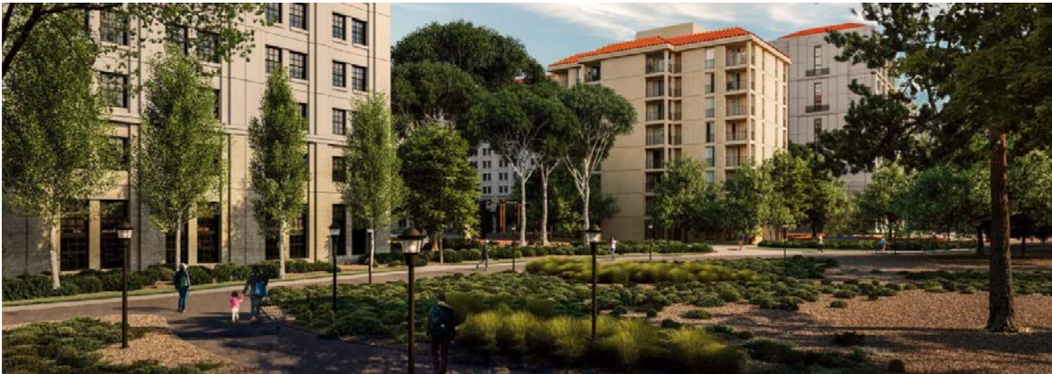
Figure A.4. Image of Escondido Village Graduate Residences (Source: Stanford Residential & Dining Enterprises Website)
