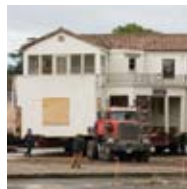
ROGERS, MARIPOSA AND SERRA HOUSES ARE MOVED TO NEW LOCATIONS IN PREPARATION FOR CONSTRUCTION OF THE MUNGER GRADUATE RESIDENCES.
